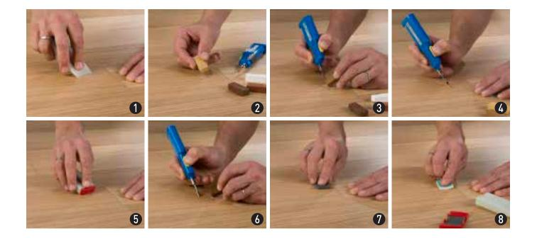
**O PREPARING**: The area to be repaired has to be clean, dry and free from grease. If necessary, remove any loose or sticking out particles with a pointed item.
